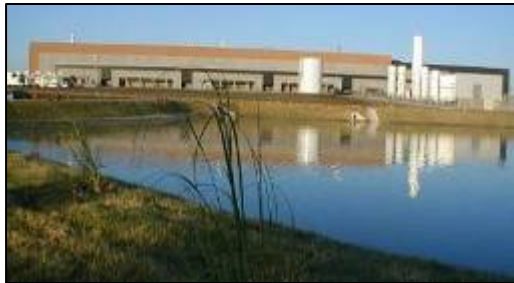
Rain Water Reuse Pond
